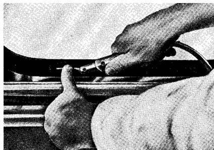
The eyelet and filler are then slipped into the appropriate channel in the glazing section but not at its joint position. The end of the filler section is held in its groove by pressure applied by the thumb of your left hand, while the eyelet is guided continuously along the edge of the window. The filler automatically slips into the groove of the sealing section thus ensuring firm connection, pre-tension and sealing.
